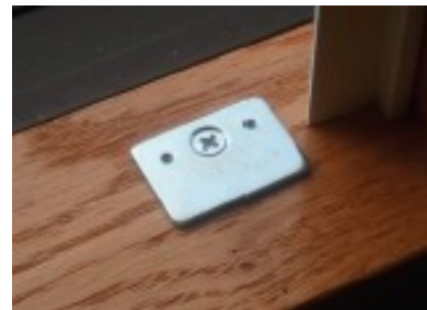
Figure 2: Strike Plate on window sill
